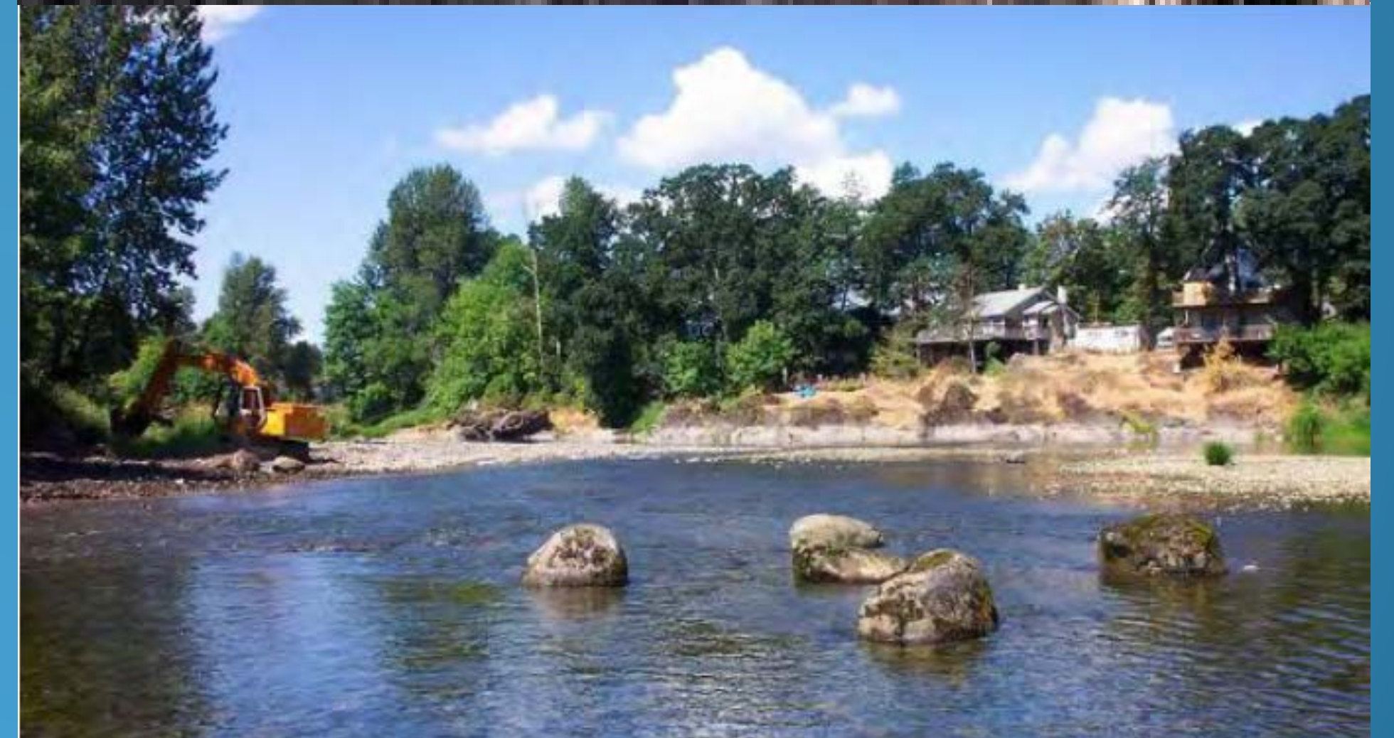
Boulder Placement ( https://www.wou.edu/.../restoration/WA_Dept_Forestry_2004_Boulder_Clusters.pdf )
