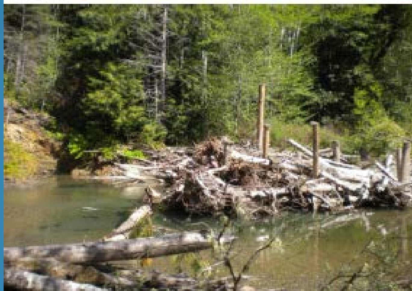
Large Woody Material - Example of ELJs on the Klamath River (USFWS 2016)
