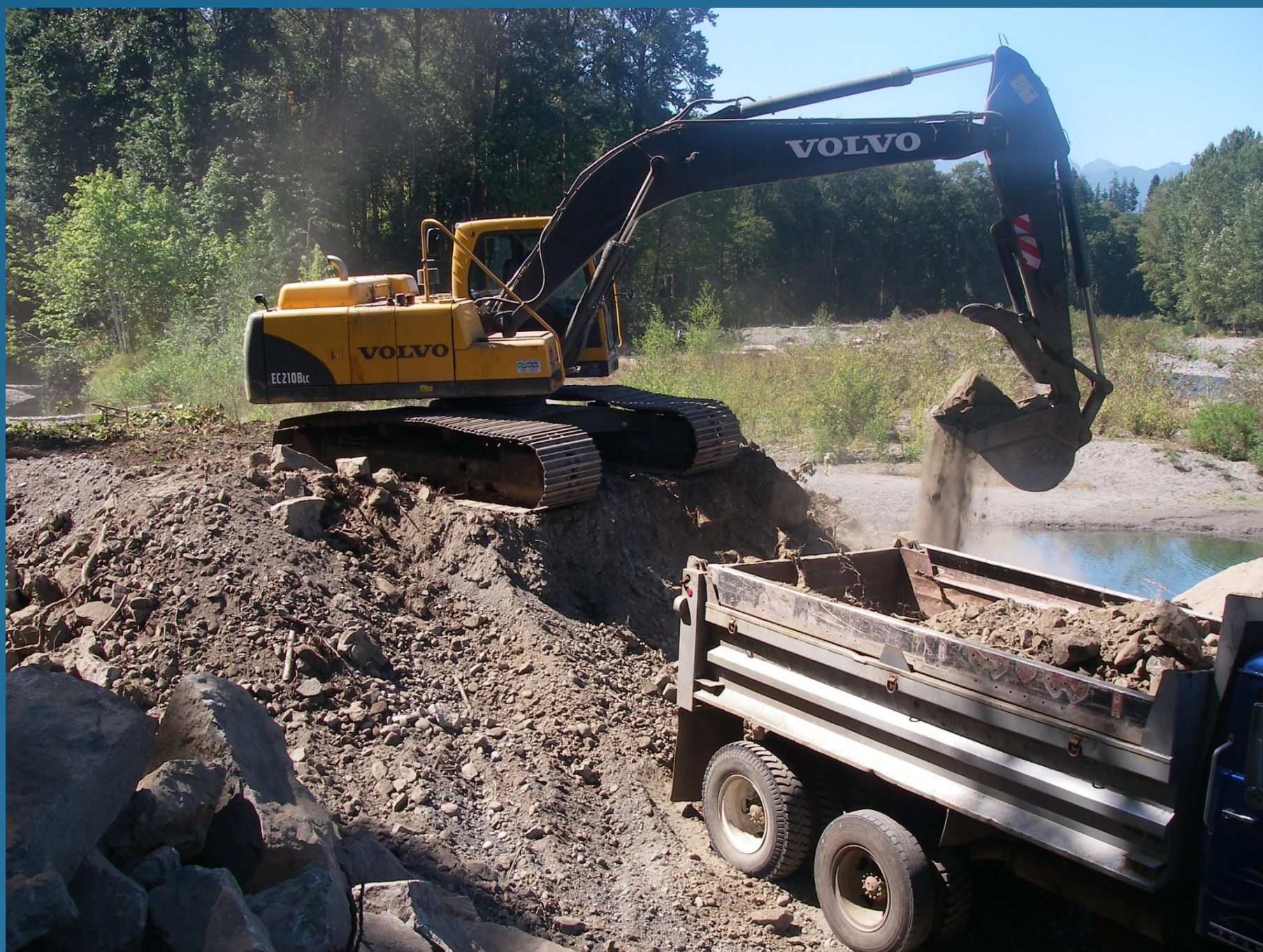
Floodplain Lowering - Lower Dosewallips Floodplain Restoration http://wildfishconservancy.org/projects/lower-dosewallips-floodplain-estuary-restoration/
